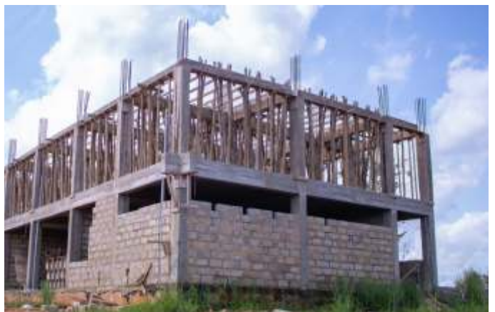
Ongoing Construction of Amenfi State University College.
