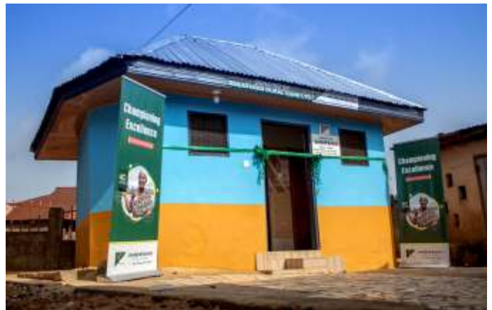
Constructed 3-Seater Washroom Facility to Bogoso Prestea Huni - Valley Education Directorate at the cost of GHC 25,000.00.
