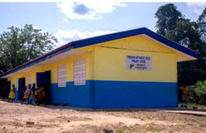
Renovated Wassa Akropong Freeman Methodist Primary/JHS.
